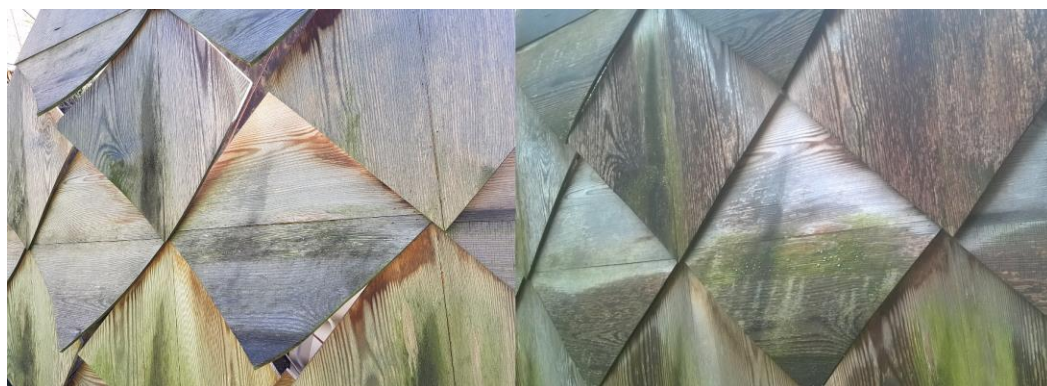
Figure 7: Ray 2 Responsive Wood Envelope Prototype a) in Semi-Dry April Weather When the Screen is Partly Open for Boundary Exchange between Exterior and Semi-Interior; b) After April Light Rain (photos: Davidová 2018 and 2017 respectively)
