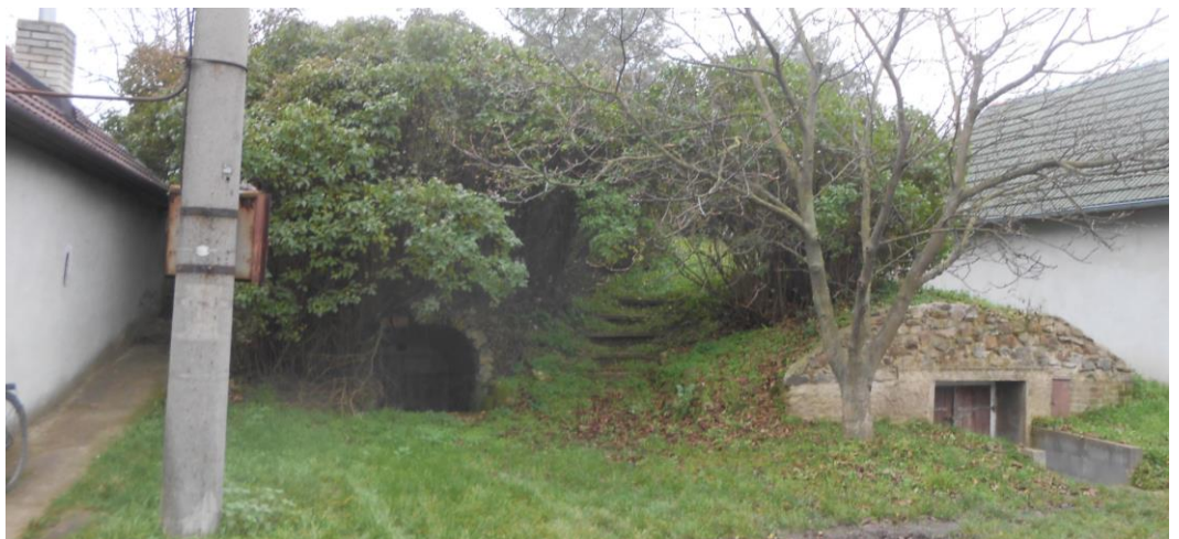
Figure 16: Combination of Subtractive and Additive Technique on Traditional Wine Cellar in Znojmo, South Moravia, Czechia. The architecture is combining such techniques with grass on the roofing and algae on the inside to generate constant climate for white wine fermentation in about 7-15°C (photo: Davidová 2014)
