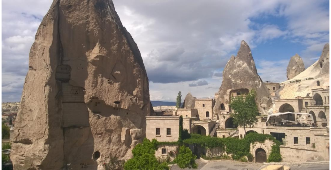
Figure 15: Combination of Subtractive and Additive Building Layers that were codesigned by variety of users for variety of seasonal use over time and cultures with different preferences in still inhabited city of Göreme by both pigeons (in front) and people (in back) (photo: Davidová 2016)
