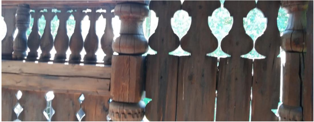
Figure 11: Breathing Envelope covering a svalgang of a store house from Nes in Hallingdal dated 1700-1797, now in Oslo Open Air Museum (photo: Raková 2017)
