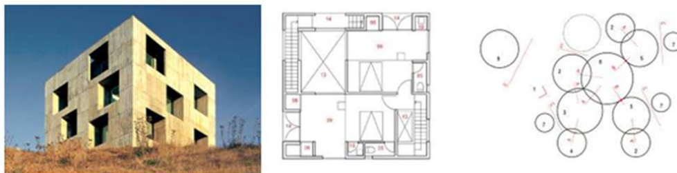
Figure 1. Casa Poli in Coliumo, Pezo von Ellrichshausen Architects (Chile, 2005). Source: Personal communication with authors (2008).
